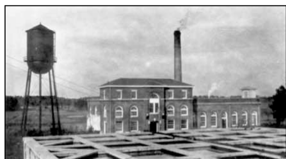
Durham City Water Works. Hillandale Plant. 1926. Finished filter system and original pump house.
